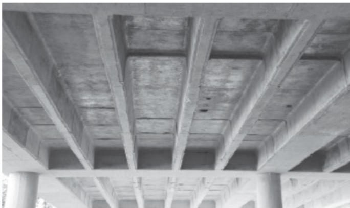
(b) Section X-X joist floor system
