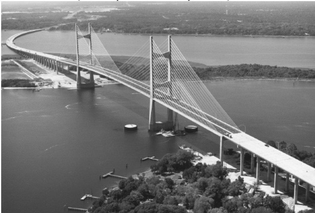
Napoleon Bonaparte Broward Bridge, with a 1300 ft center span at Dame Point, Jacksonville, Florida. ( HNTB Corporation, Kansas City, Missouri )
